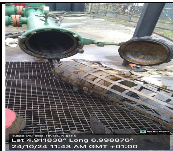
PIG RECOVERY AT RUKPOKWU MANIFOLD
