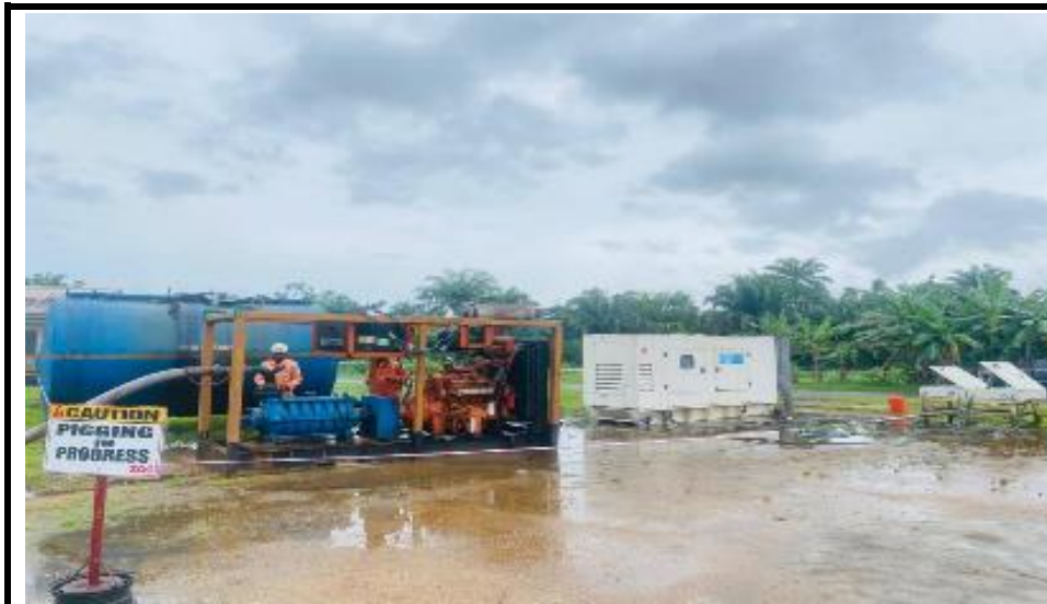
EQUIPMENT SPREAD FOR AUXILIARY PUMPING SUPPORT
