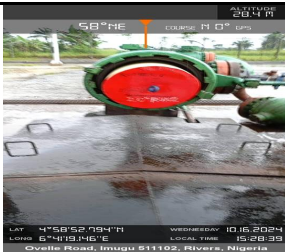
LOADED 20" MD BARE BODY FOAM PIG (RUN 2)
