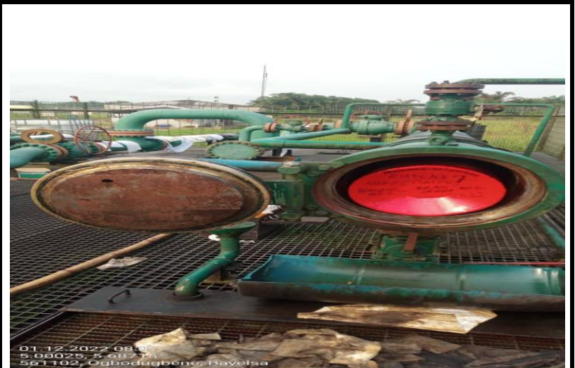
LOADED 12" MD BARE BODY FOAM PIG (RUN 7)
