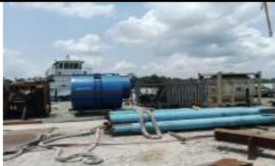
EQUIPMENT SPOTTED AND POSITIONED
