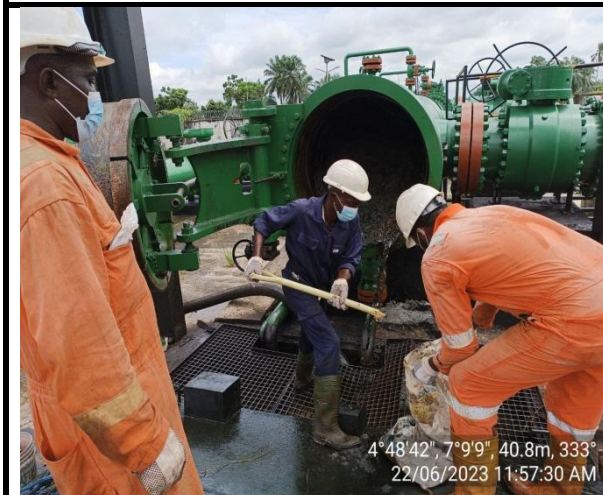
EVACUATION OF DEBRIS FROM THE BARREL
