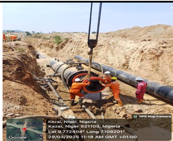
LOADING OF MANDREL PIG
