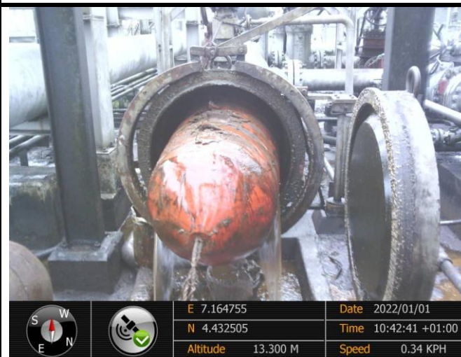
24" MD COATED FOAM PIG RECOVERY @ BONNY OIL GATHERING TERMINAL (BOGT)
