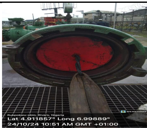
PIG RECOVERY AT RUKPOKWU MANIFOLD
