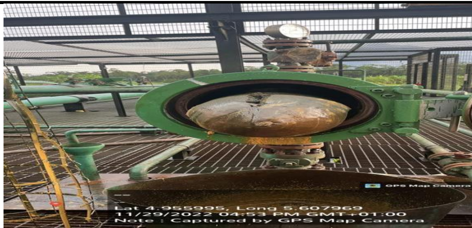
12" MD MD FOAM PIG AT THE RECIEVER BARREL
