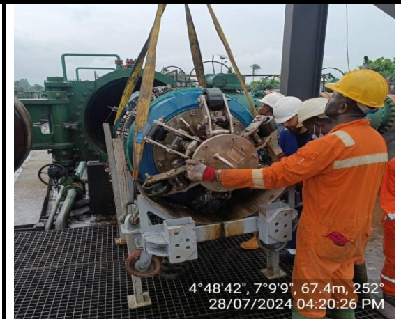
RECOVERING OF INTELLIGENT PIG AT OGALE MANIFOLD
