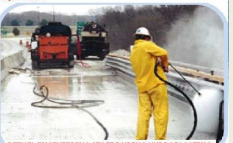
BETHEL ENGINEERING STAFF DURING HYDROBLASTING OPERATION
