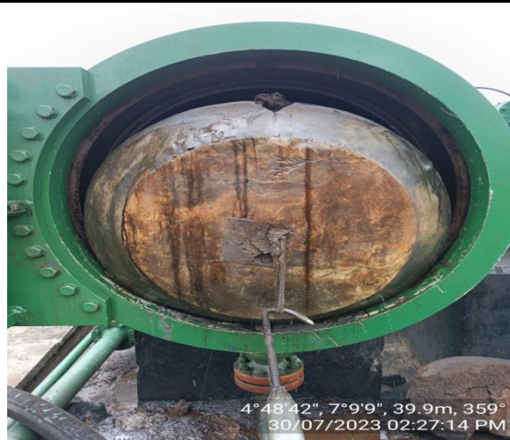
RECOVERING OF 36" DEWATERING PIG
