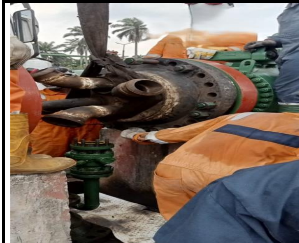
INSTALLATION OF HOOK UP POINTS
