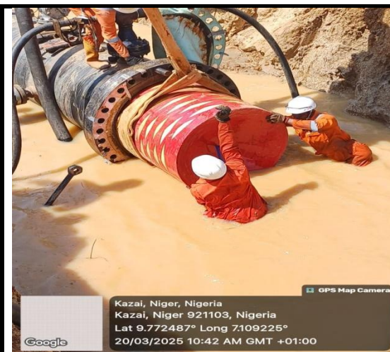
LOADING OF 40" MD COATED FOAM PIG
