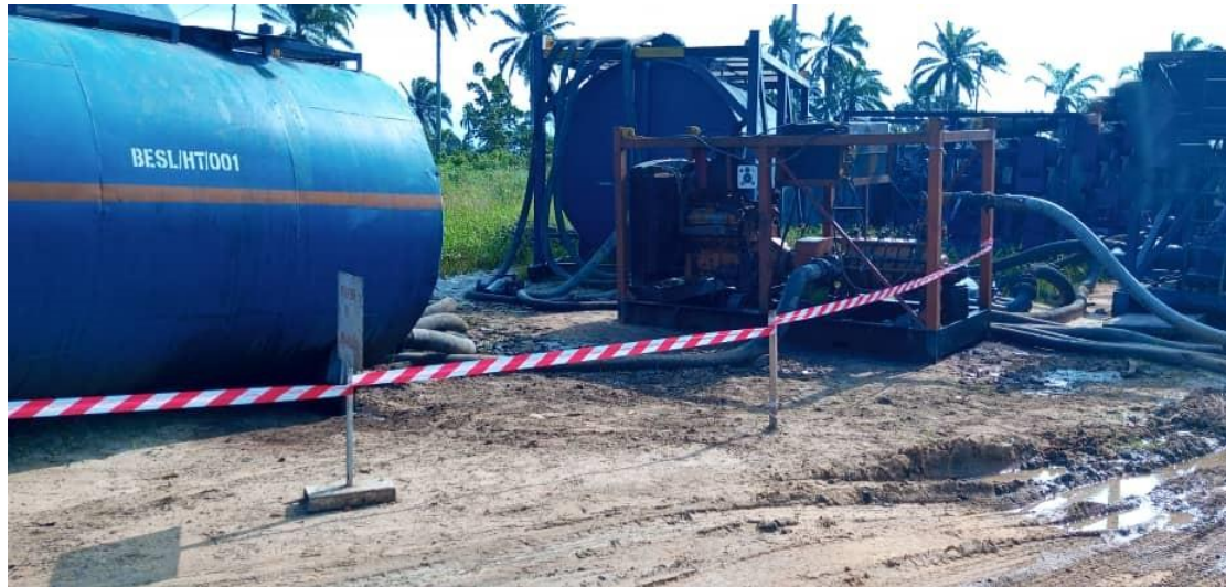
EQUIPMENT SPREAD FOR AUXILIARY PUMPING SUPPORT
