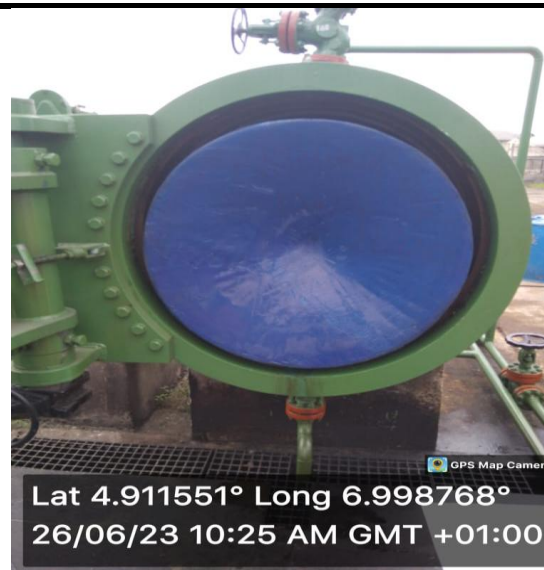
LOADED 36" MD COATED FOAM PIG (RUN 2)
