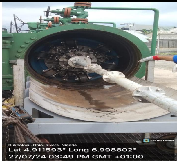
LOADING OF INTELLIGENT PIG
