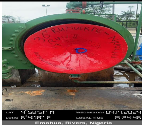
LOADED 36" MD BARE BODY FOAM PIG (RUN 2)
