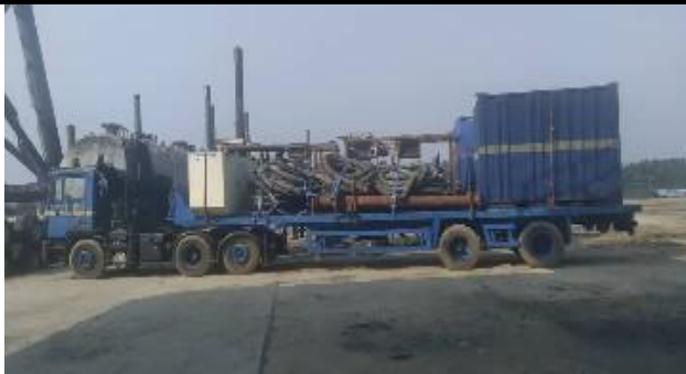
EQUIPMENT MOBILIZATION FROM BASE TO WORK SITE
