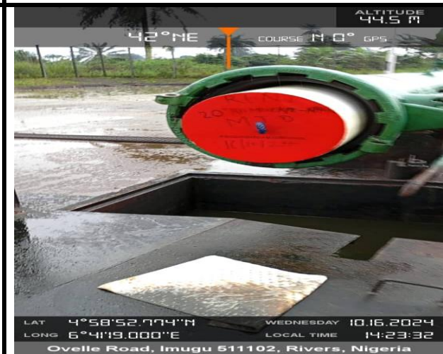
LOADED 20" MD BARE BODY FOAM PIG (RUN 3)
