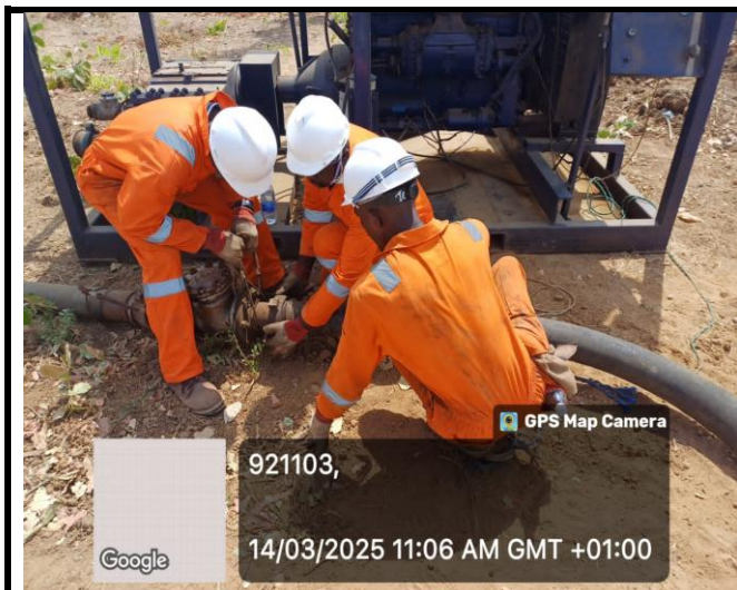
EQUIPMENT RIG UP ONGOING
