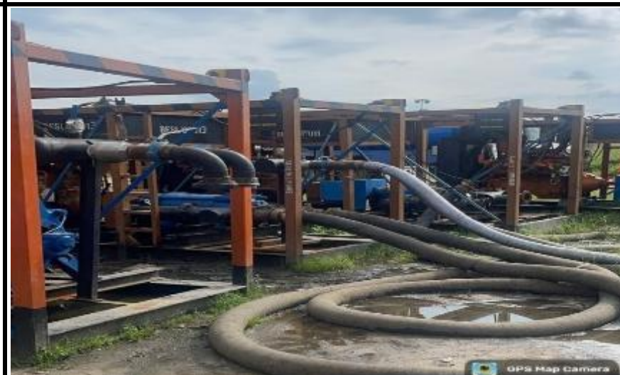
PUMP SPREAD FOR AUXILIARY PUMPING SUPPORT
