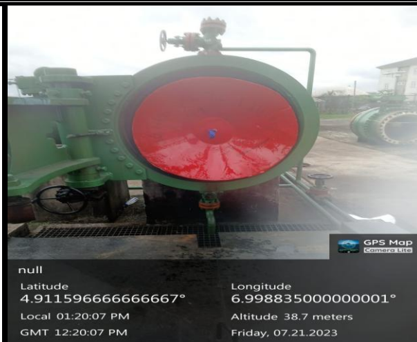
LOADED 36" MD FOAM FLUSHING PIG RUN 1
